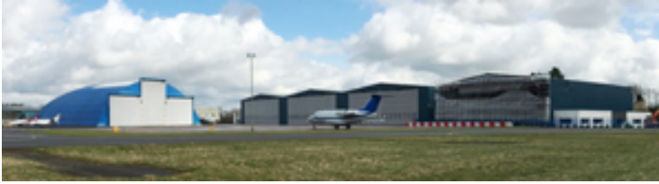
New hangar taking shape at London Oxford Airport
